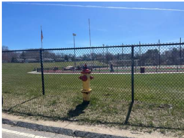
Figure 3: Hydrant near Field
