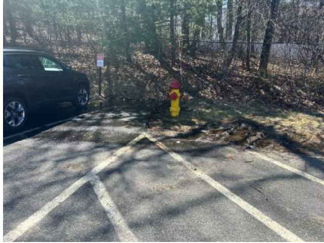
Figure 6: Hydrant South of Building
