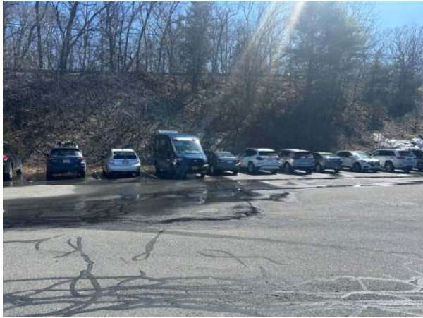
Figure 17 – Ponding at Parking Lot to South
