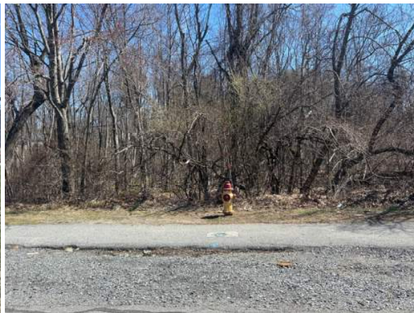
Figure 4: Hydrant on Access Drive
