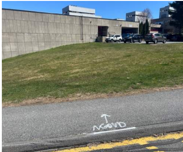
Figure 20, 21, 22 – Gas Line Dig Safe Markings in Courtyard and Parking Lot
