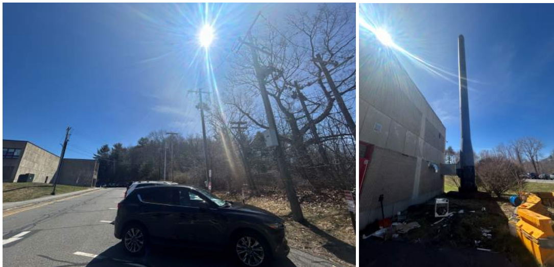
Figure 24, 25, 26 – Site Lighting, Overhead Wires and Electric Manhole
