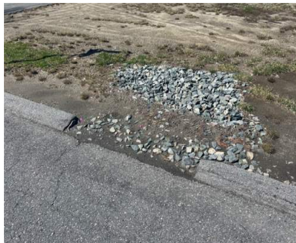
Figure 24 – Stone Drywell or Inlet
