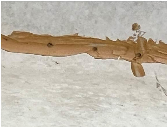
Example of past repairs to the flanges and stems of the precast concrete double tees
