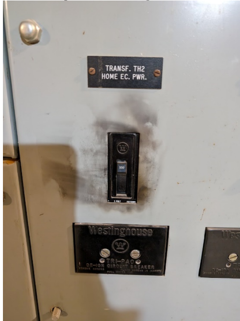
Figure 1 Switchboard 1 Fire Damage
