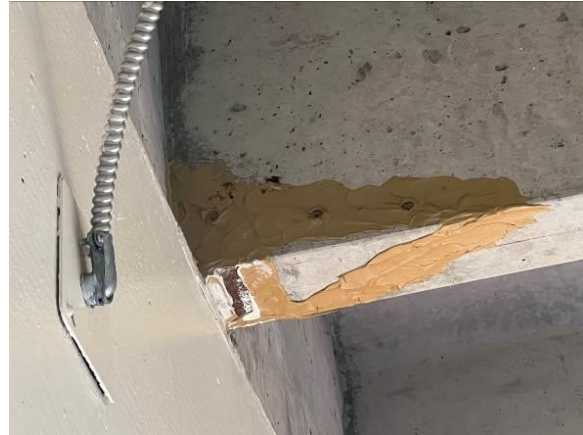
Example of past repairs to the flanges and stems of the precast concrete double tees
