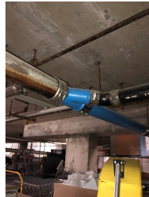
Photo 12 – Polypropylene Piping
